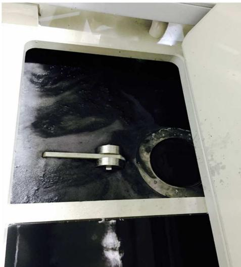
**Floating skimmer within a degreasing tank**
